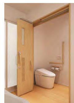
A sliding door with sufficient width to allow for easy access by wheelchair and care workers.
