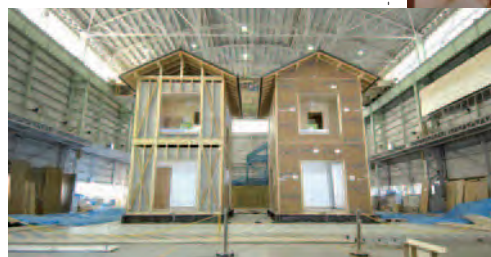
Exterior wall base material Dailite (durable surface material)
